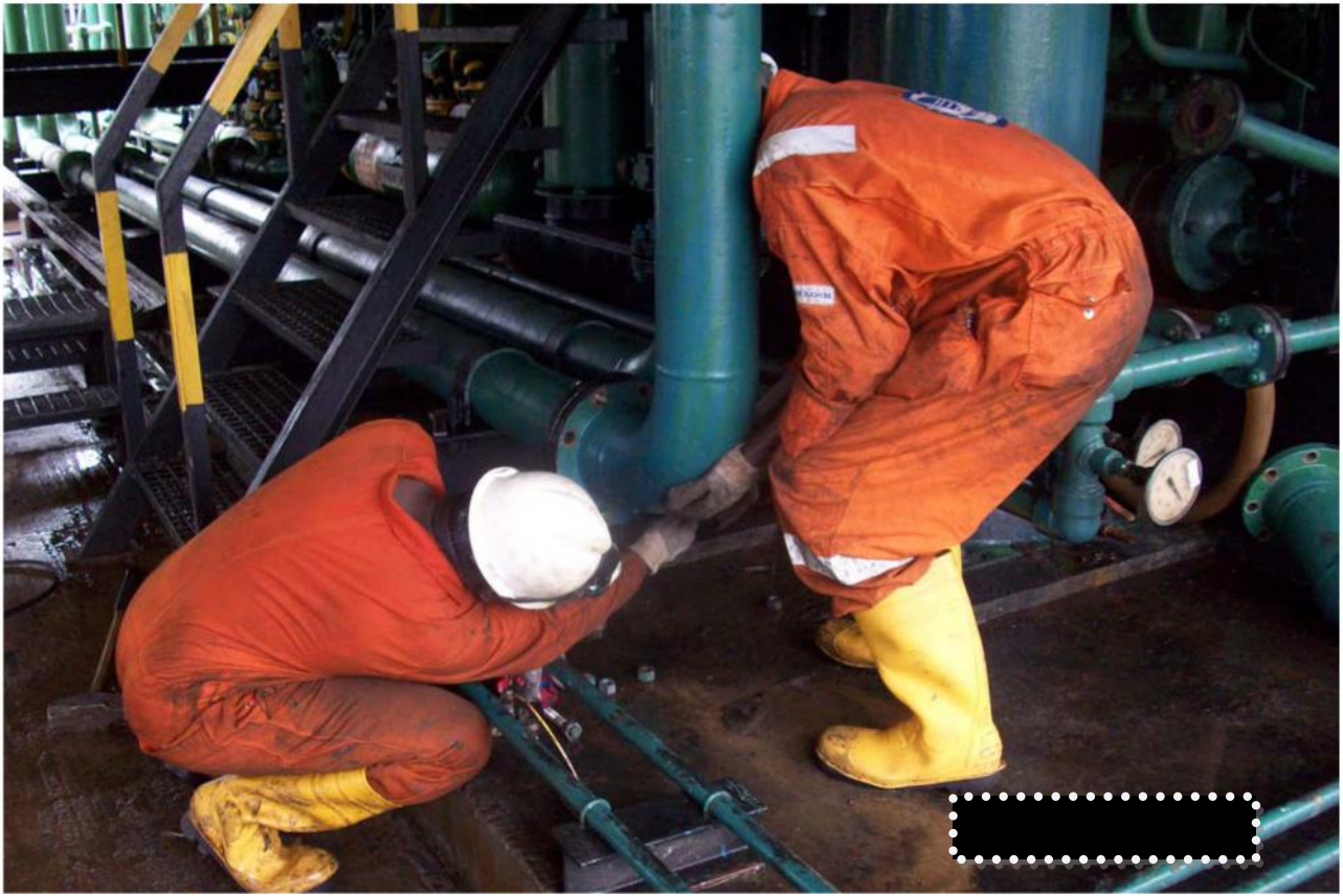
Process line cleaning and chemical cleaning of process pipes.
