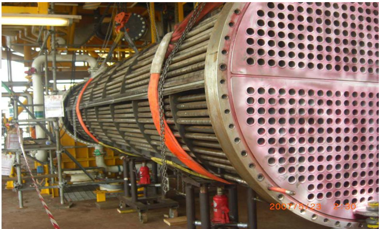
Inspection of tube exchanger
